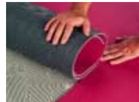
Step 3: Unroll the rubber flooring over the adhesive.
