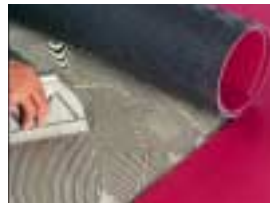
Step 2: Apply recommended adhesive to the Everlay surface.
